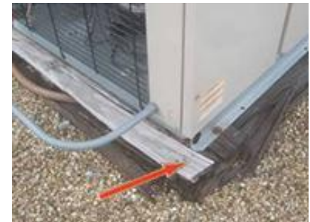
DAMAGED CURBING
