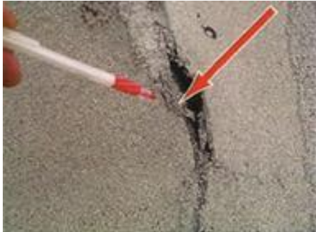
FAILED FLASHING
